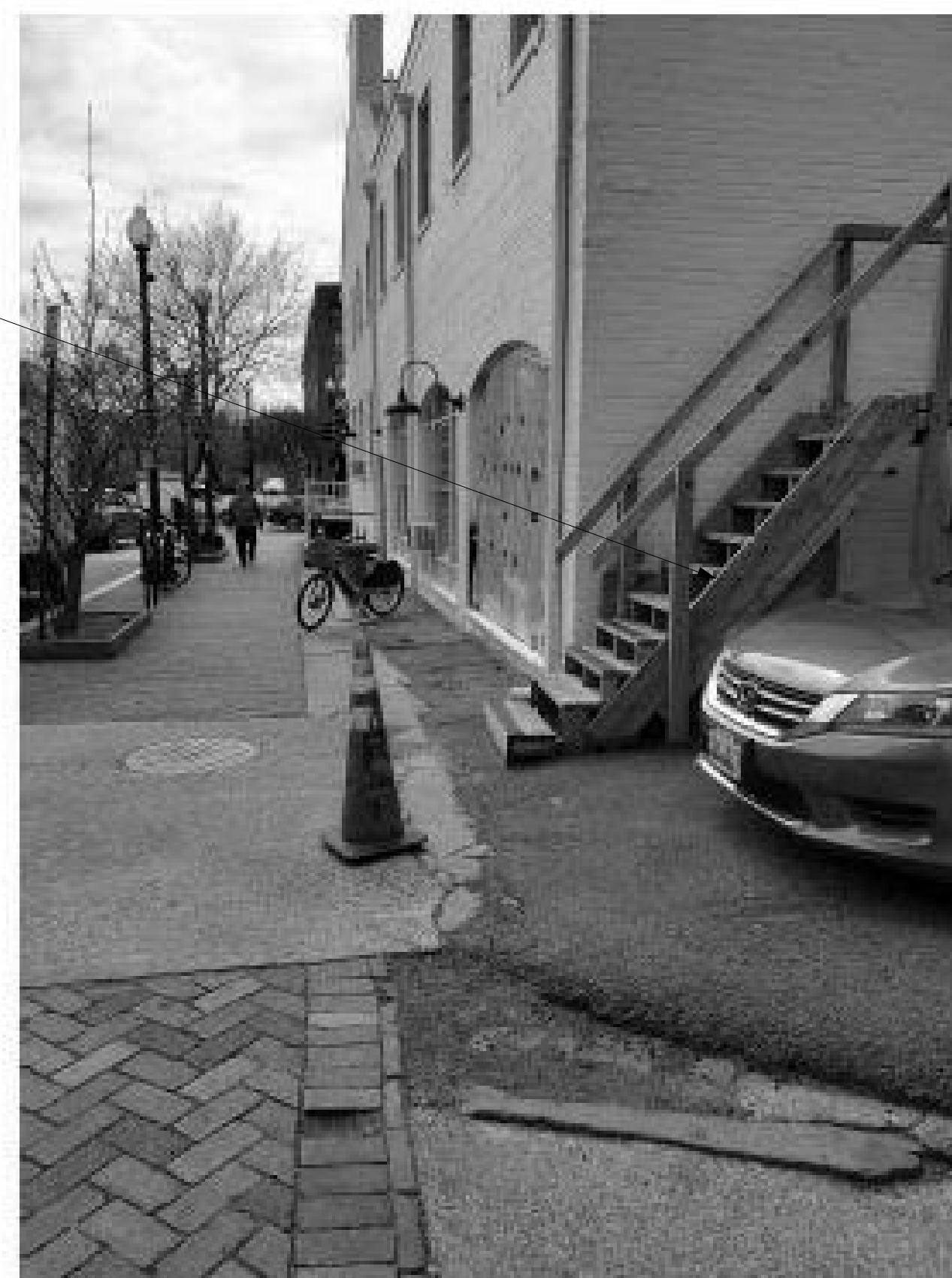
Existing Side/Rear 2805 M St.
