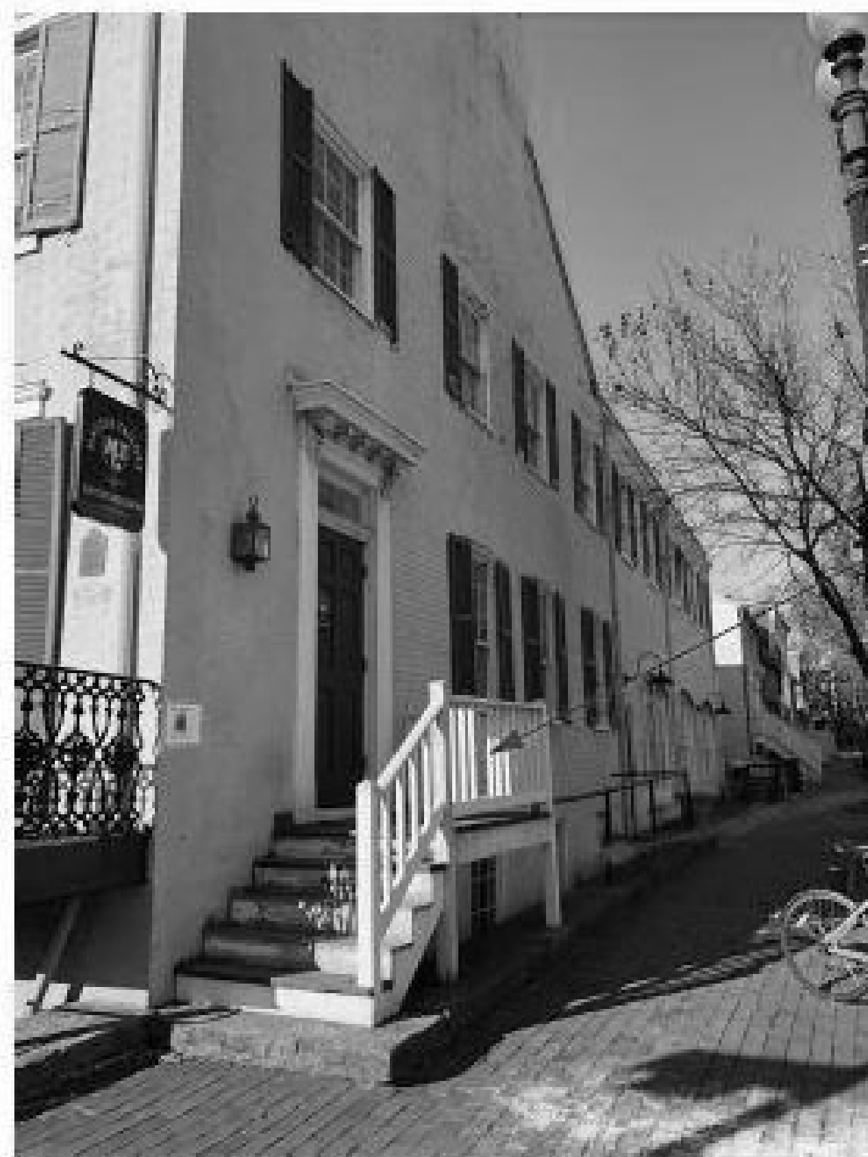
Existing Side 2801 M St.
